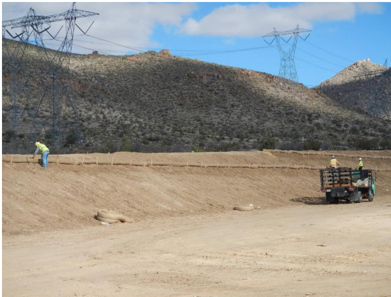
Photo 8: BMPs consisting of straw wattles were observed being placed along slopes at the ECO substation site in accordance with the SWPPP and MM-HYD-1.
