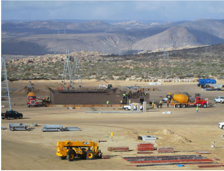
Photo 7: The control shelter at the ECO substation was observed being constructed with an Otay Ranch Brown-colored split face concrete block in accordance with the Surface Treatment Plan and MM-VIS-3g.
