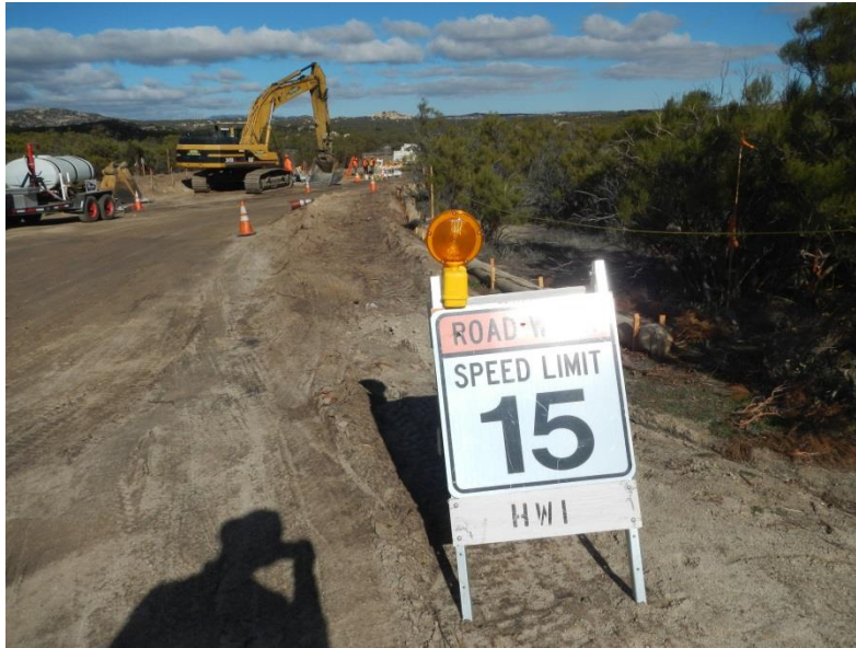
Photo 3: In accordance with MM-BIO-7b, speed limit signage is posted along access roads during construction of the 138 kV underground alignment. Construction vehicles are not to exceed 15 miles per hour on unpaved roads and the right-of-way accessing the construction site.
